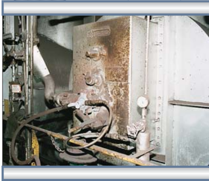
The burners are installed on existing equipment.
